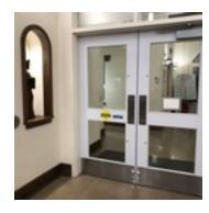
2. The doors were carefully tested, so that a person pushing a wheelchair can trigger the button six feet prior to the door, which allows the doors to open, and roll through, without a dance of approaching the door, rolling forward and back to provide clearance to enter.
